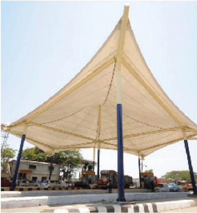
IRB Toll Plaza, Bhiwadi
