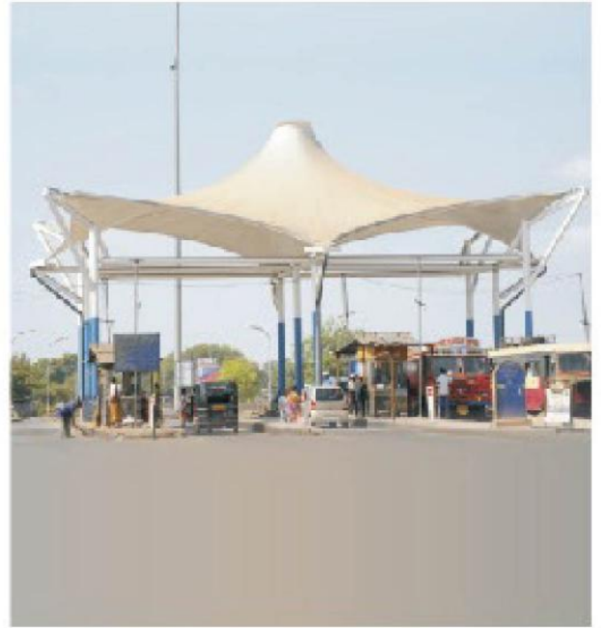
IRB Toll Plaza, Kharpada
