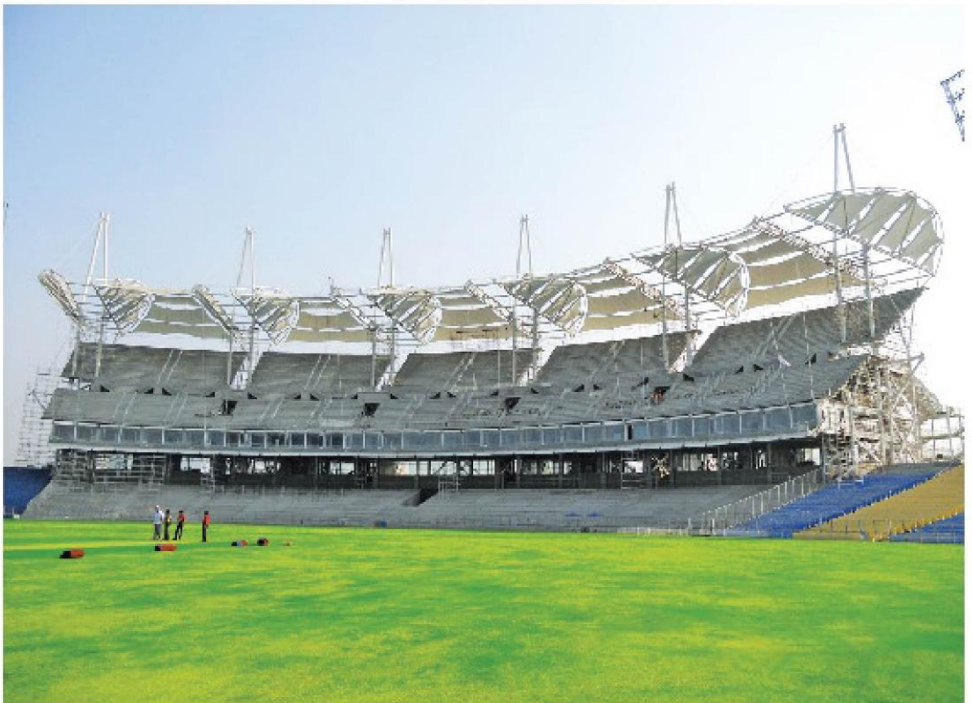
Cricket Stadium, Pune
