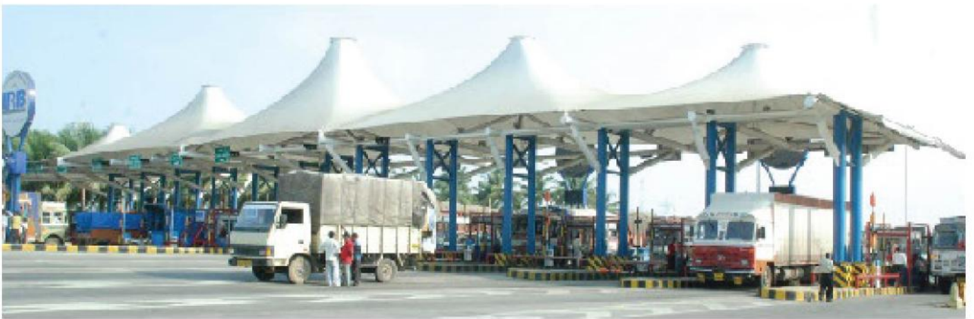
IRB Toll Plaza, Bharuch
