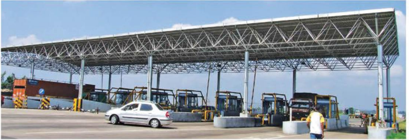
Toll Plaza, Kolhapur
