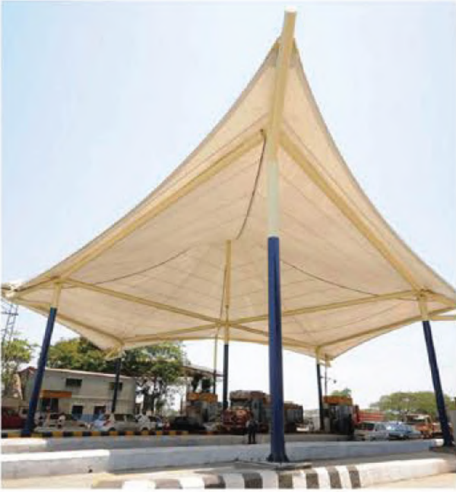
IRB Toll Plaza, Bhiwadi
