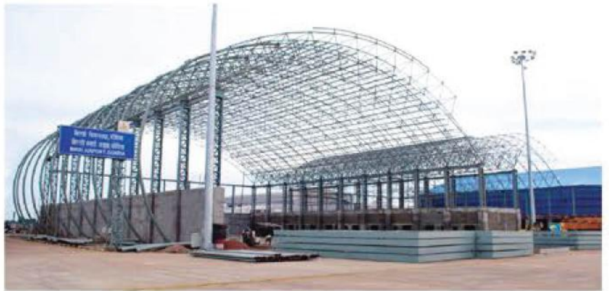
Airport Hangar, Gondia
