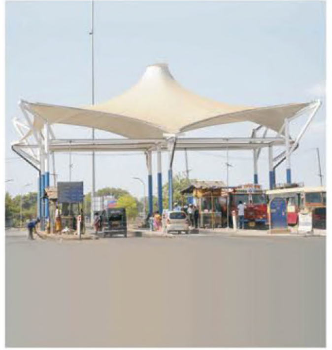
IRB Toll Plaza, Kharpada
