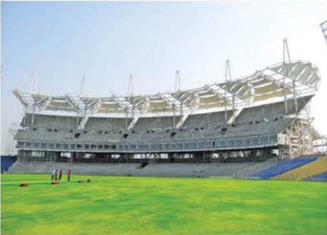
Cricket Stadium, Pune
