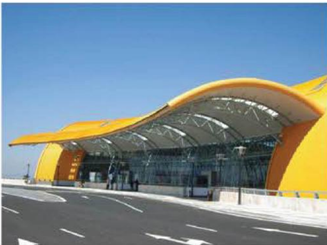
Lien Koung Airport Terminal Building
