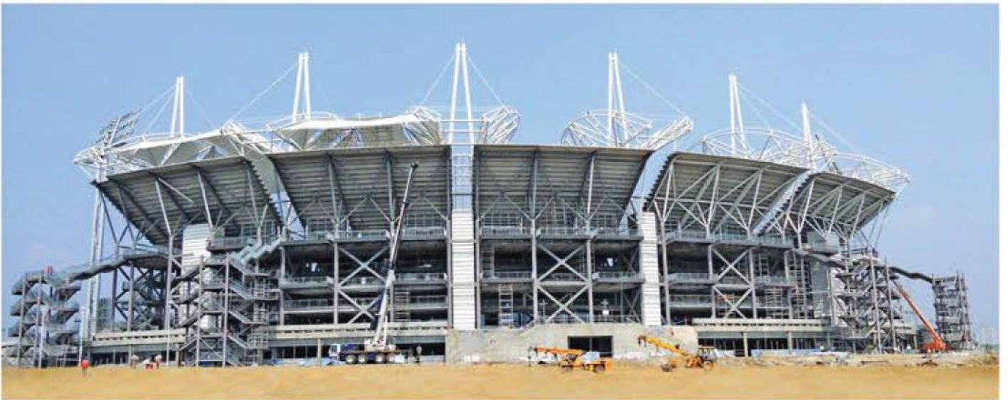
Cricket Stadium, Pune
